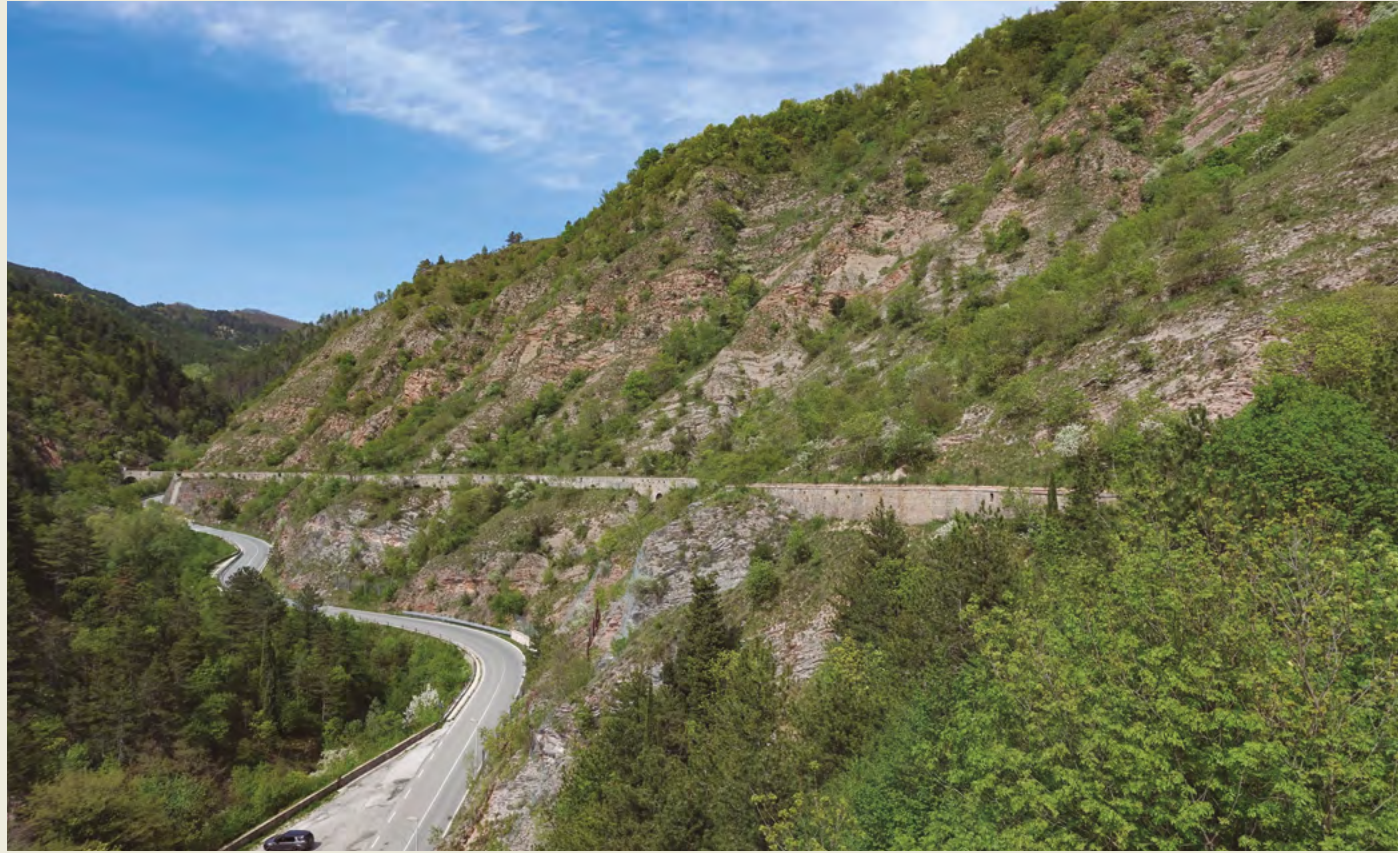
Upper part of the Bottaccione Gorge section, showing the Campanian and Maastrichtian part of the section. A medieval aqueduct is also seen. (Photo by Birger Schmitz).
