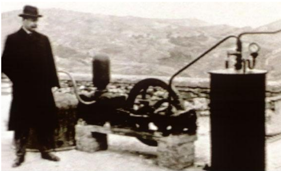
First Geothermal Power Plant, 1904, Larderello, Italy
